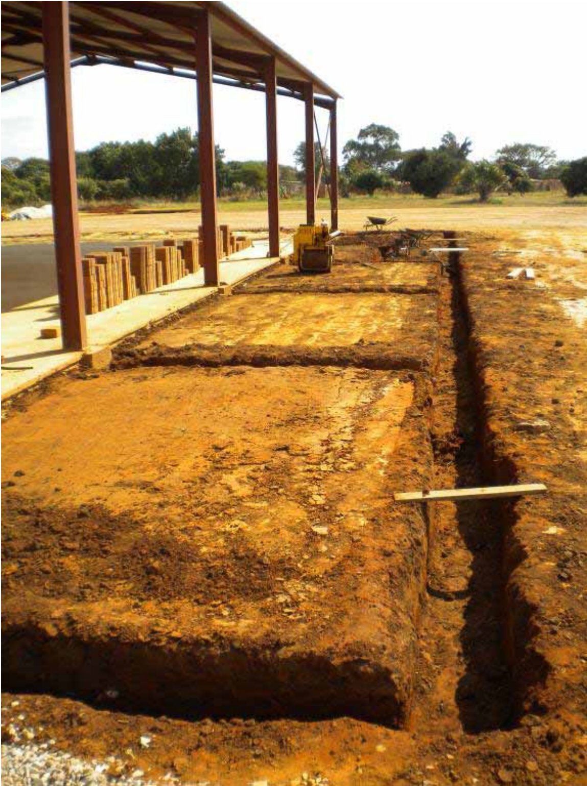
Before concrete and setting up the form work.
